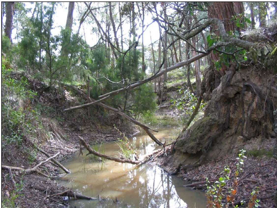
Figure 2.6. Feature WF38 revegetated but still active gully erosion, north of Invermay.
