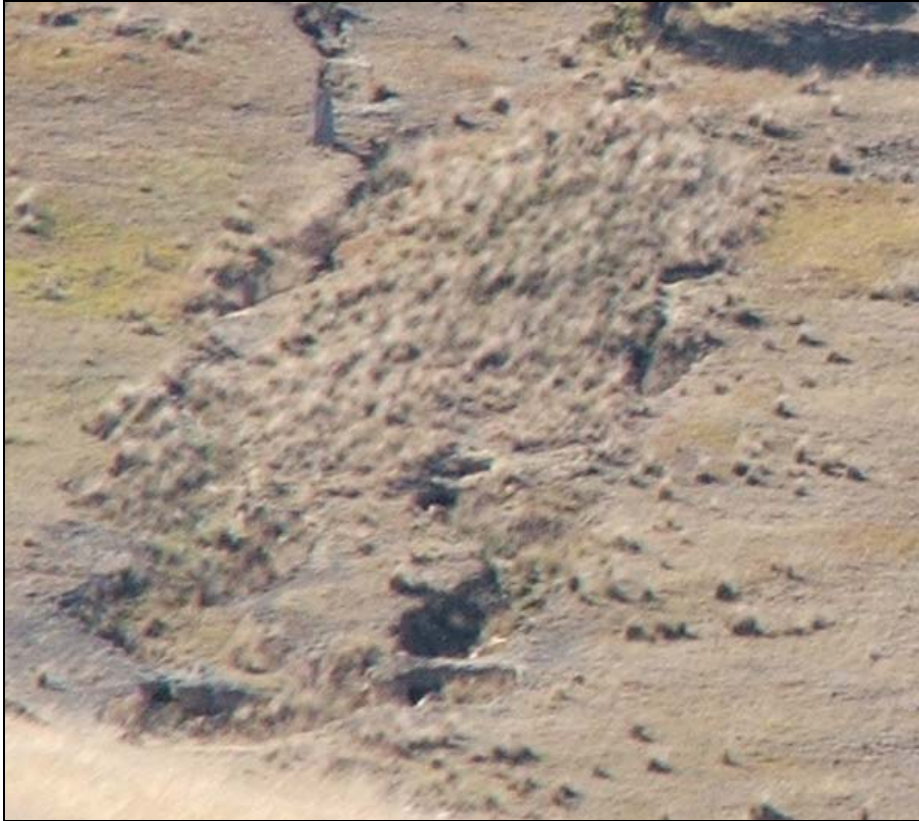
Figure 2.8 Feature WF2427. Tunnel erosion south of Berringa.
