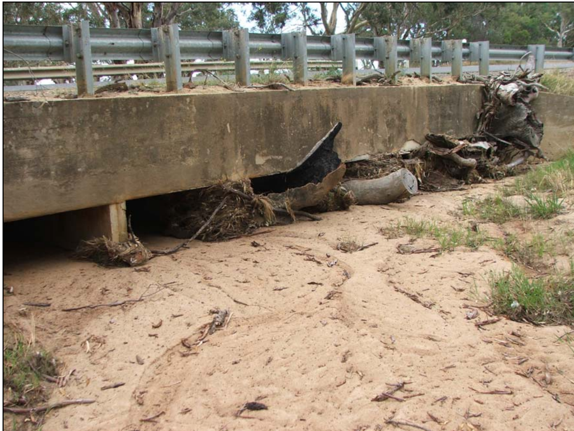
Figure 2.11 Feature WF2398. Stream sediment obstructing a road bridge along the Geelong - Bacchus Marsh Road.
