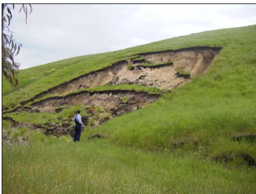
Figure 2.4 The Moorabool landslide, 2001
