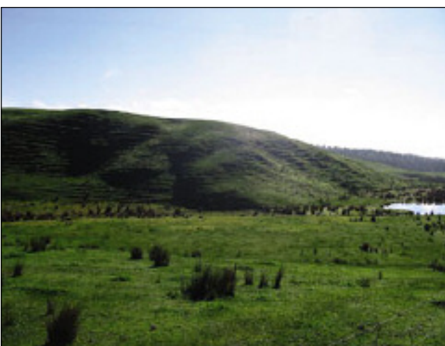
Figure D4: Landslides adjacent to Scrubby Creek (Upper Barwon Landscape Zone) Photograph: A. Miner 2006
