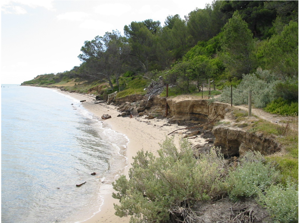
Figure B 17 Coastal foreshore erosion and degradation at Clifton Springs.
