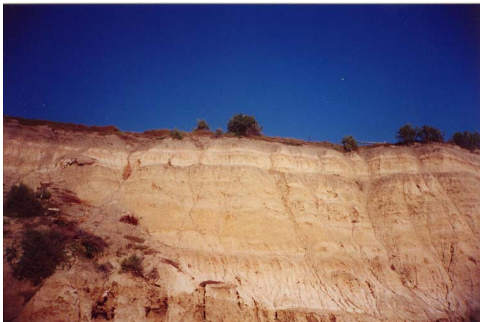
Figure B 6 Sheet and rill erosion below Beacon Pt Rd, Clifton Springs.
