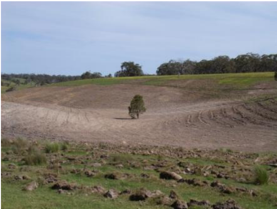
September 2007: After photo showing entire gully works completed and using the blackwood tree for positioning. Note surrounding slopes have been ripped ready for planning.
