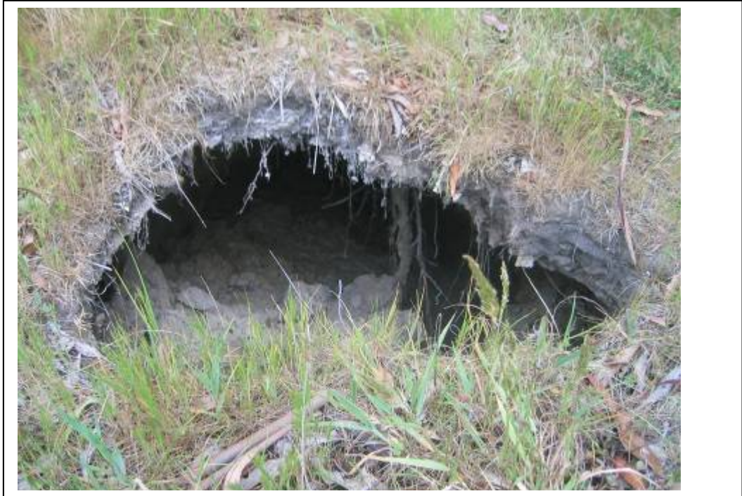
Photo 5 November 2006, a section of the track has re-collapsed, opening up a 2m sq. 'cave' under the area previously worked on.
