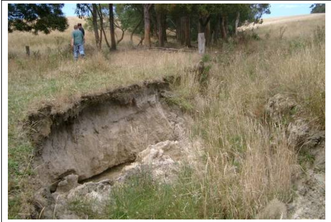
Photo 1 Initial site assessment prior to works February 2005. Photo taken looking east
