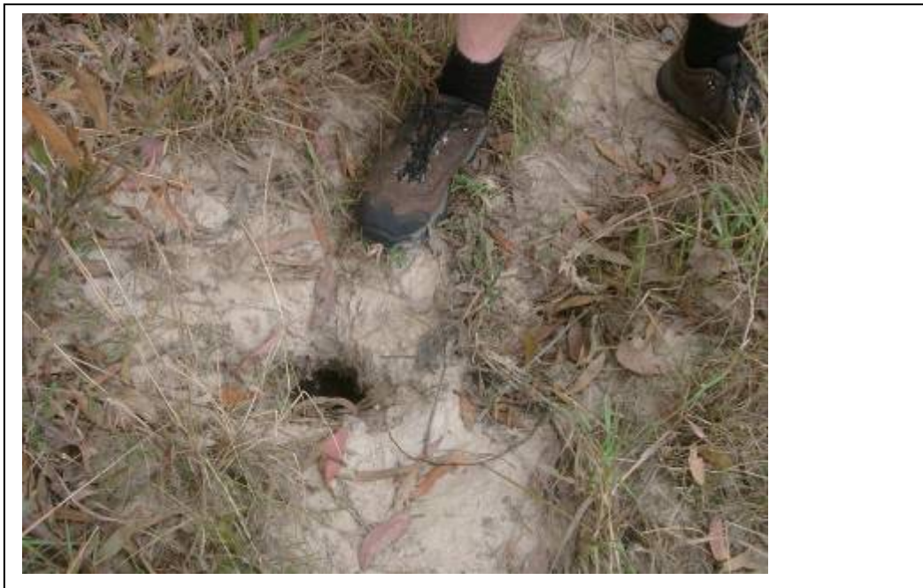
Photo 5 November 2006, a section of the track has re-collapsed, opening up a 2m sq. 'cave' under the area previously worked on.
