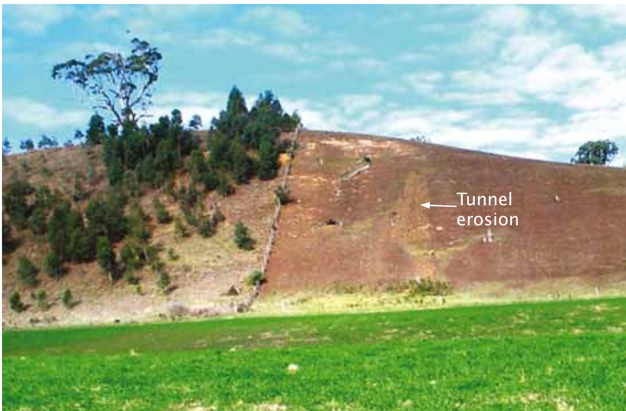
Left of the fence has been revegetated with indigenous species and right of the fence has not been rehabilitated. Note the lines of sediment from the working tunnel erosion on the right.
