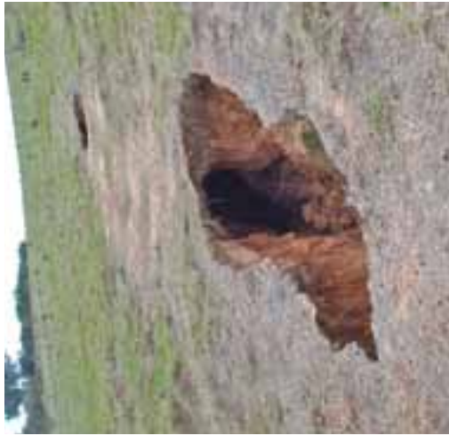
Figure 2: Partial collapse of tunnel with drying off lines visible.
