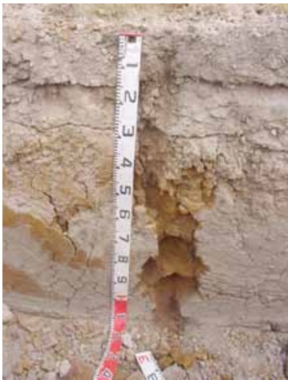
Figure 24: Cracks in the soil that lead to tunnel erosion.
