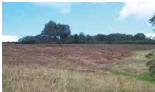
26b Glenaladale paddock during treatment with heavy machinery.
